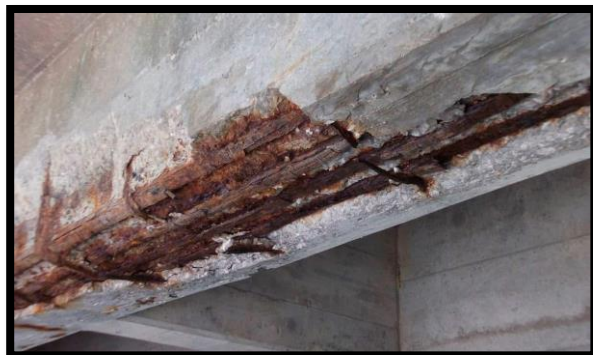
Figure 37: Corrosion of Steel Reinforcement
