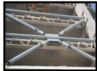
Figure 74: Shock Absorbers
