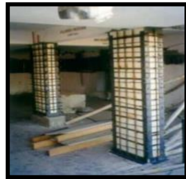
Figure 78: Jacketing of Column
